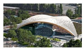
The Pacific National Exhibition (PNE) has unveiled the design for its new amphitheatre which includes the largest free-span timber roof structure in the world.
